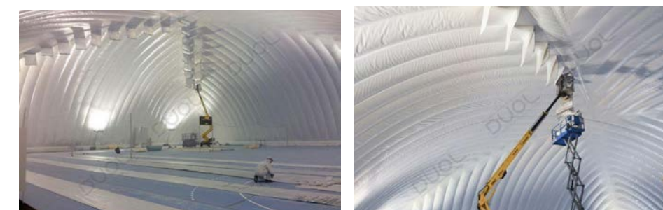
DF Ultra Insulation during installation.
